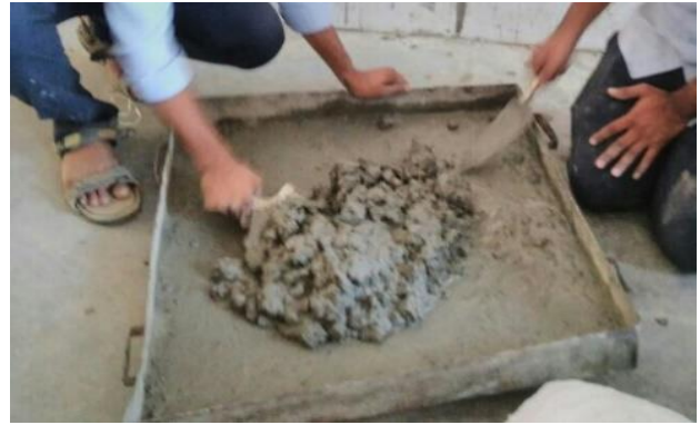
Fig (2.2) Preparation of Concrete Mixing
