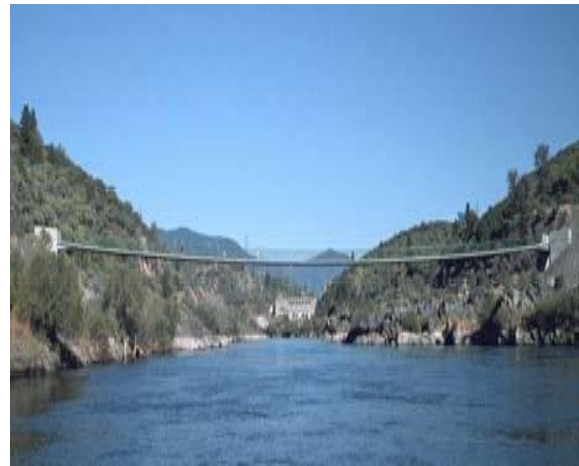
Fig. 1 Redding Pedestrian stress ribbon bridge.
