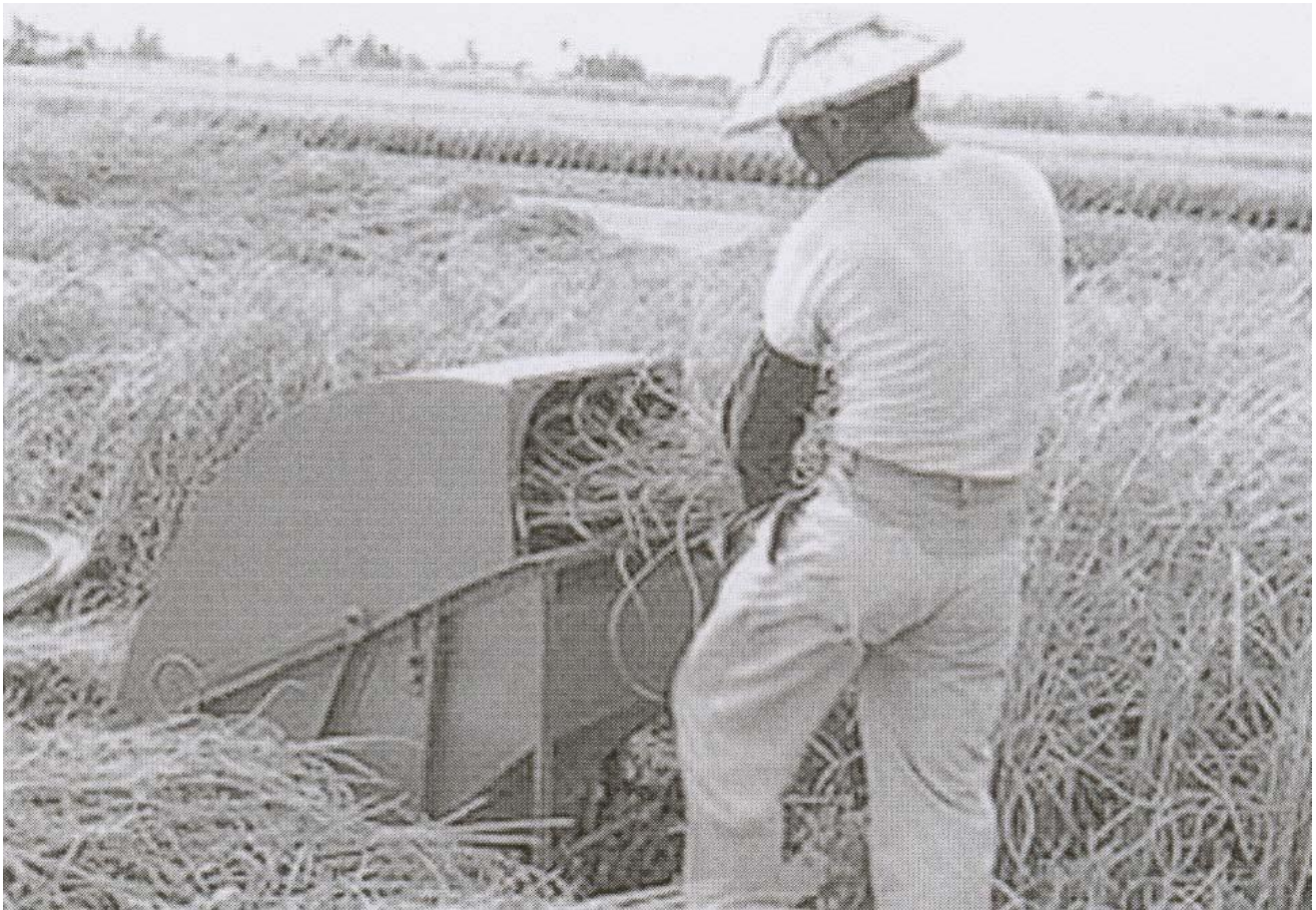
Figure 2. Small Pedal Operated Rice Thresher
