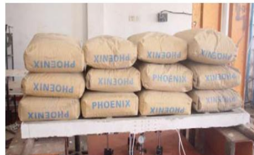
Precast layer test set-up for uniformly distributed load Summary of Theoretical and Experimental results
