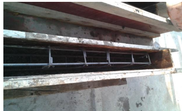
Fig3.3: Formwork for beams
